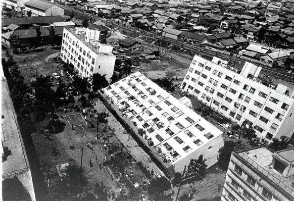
Apartments in Niigata City after the earthquake, June 16, 1964
