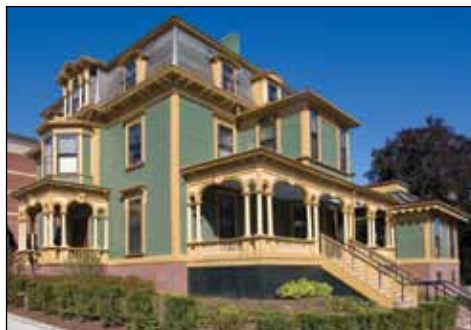
BELOW Peter Green House 79 Brown Street
